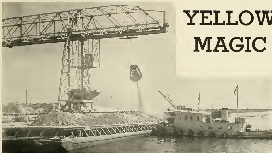
Unloading Sulphur from Barge to Vat, Port Sulphur, La.
